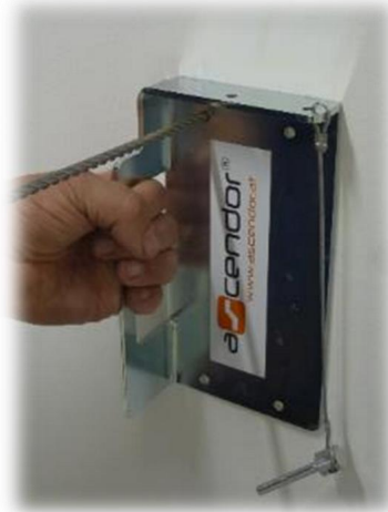
Once location of housing has been selected, hold template to wall and drill first hole. (Ø6mm)
