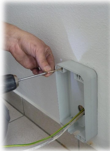
Once location of housing has been selected, hold template to wall and drill first hole. (Ø6mm)
