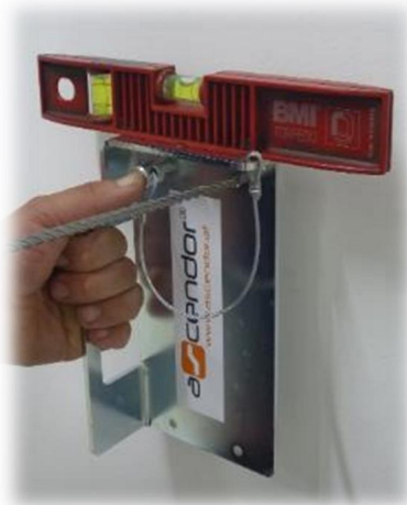
Drilling Templates for recharger housing (right) and wall mounted operating unit (left)
