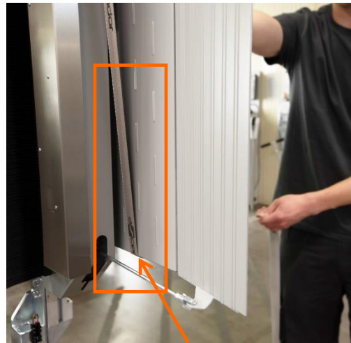
Insert the tension belt between platform and threaded rod at the bottom of the lift.
